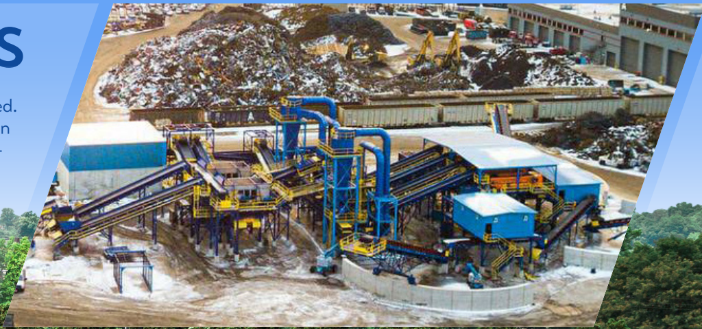
400+ TPH Ferrous Cleaning System (Low Copper)
