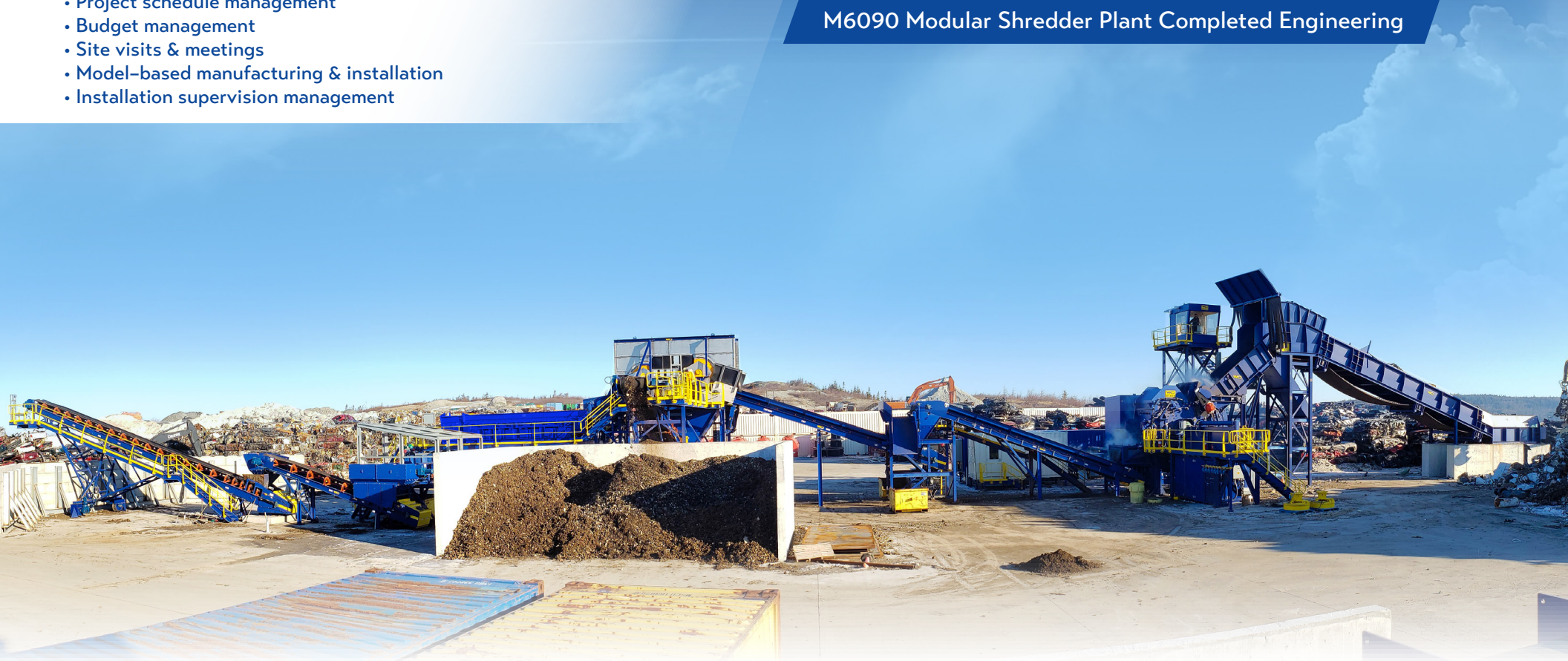
M6090 Modular Shredder Plant Installed
